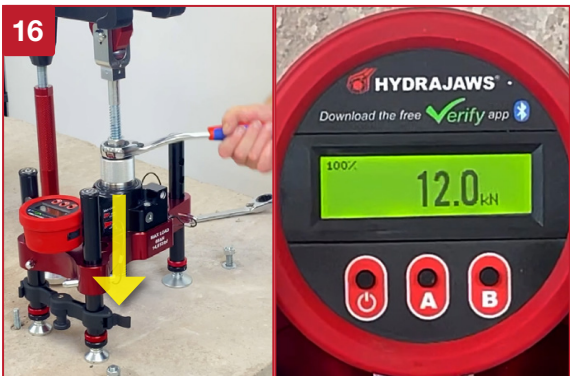
Use a ratchet spanner to test to a max of 12kN (according with your Davit Base specifications).
